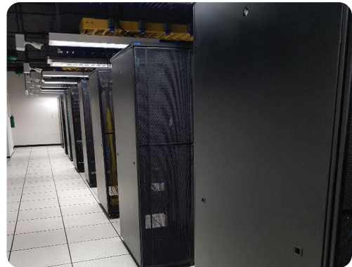
Double floor, raised floor to prevent water leakage that may cause damage to computer equipment
